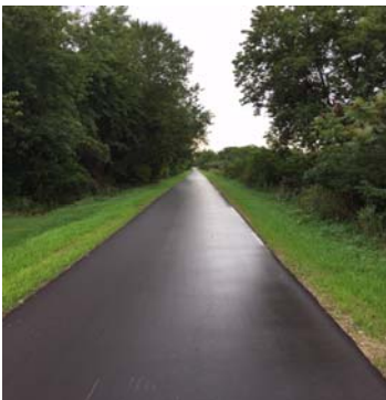
Looking for a smooth ride, the newly repaved Hart-Montague trail
