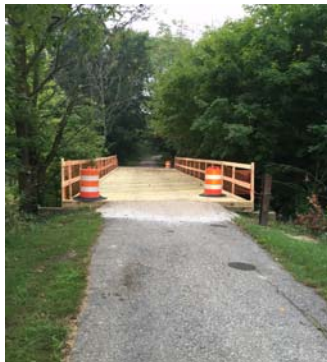
Trestle that was replaced on the Hart-Montague trail
