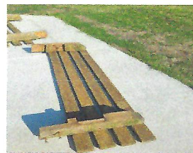
Bench before repairs
