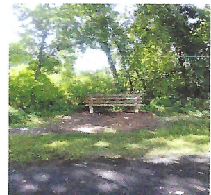
Completed bench installed
