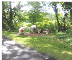
Reinstalling the bench
