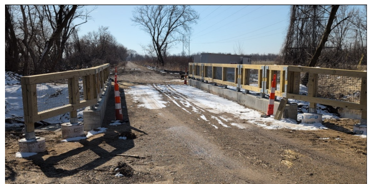
Complete culvert and handrail
