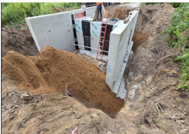
Installation of a box culvert in progress
