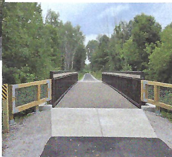
Rio Grande Bridge construction
