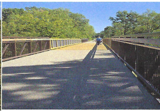
Crockery Creek Bridge Rebuild 2026
