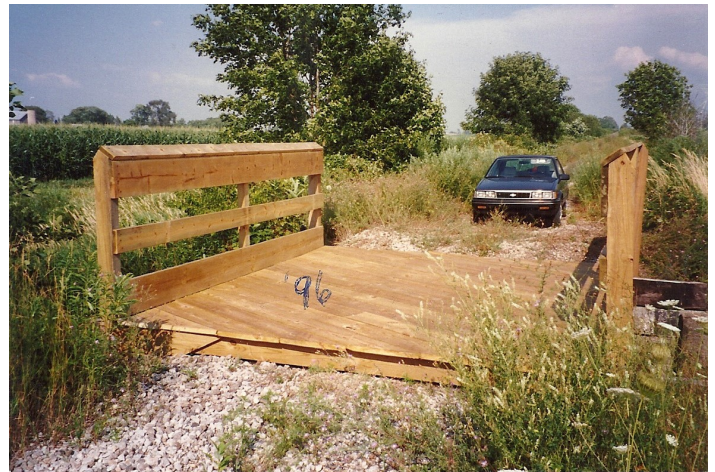
Building of a bridge in 1996
