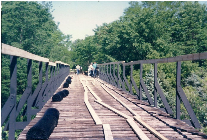
Building trestle over Crockery Creek
